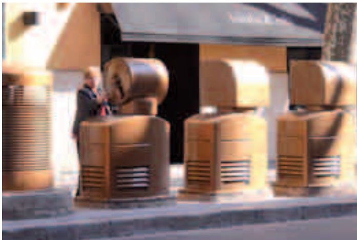
Pneumatic waste collection.
